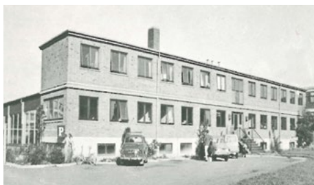
IN JANUARY 1970, BUCH & HOLM MOVED TO NEW AND MODERN FACILITIES WITH 4000 M2
